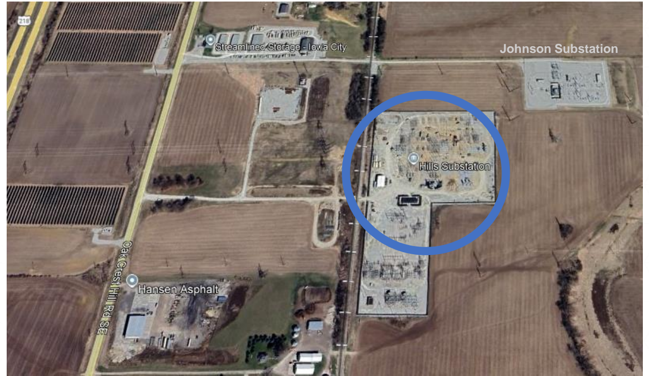
MidAmerican Energy's Hills Substation near Hills in Johnson County.
